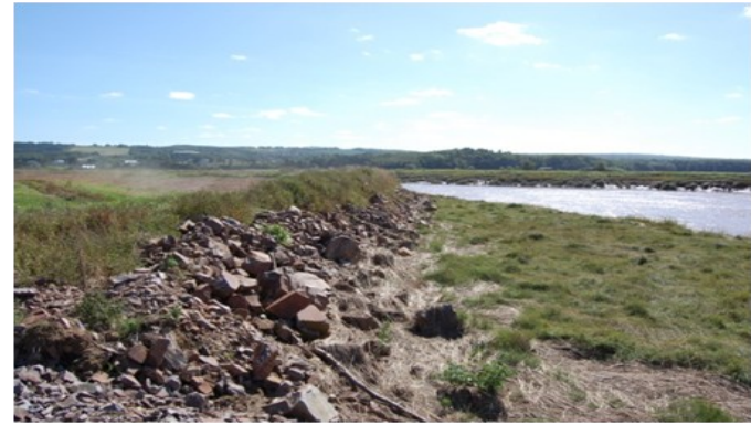
Fig3. Rock fill on the Bishop-Beckwith Dyke, Port Williams.
